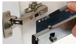
**STEP 3:** Mark the holes on the pencil line. Drill hole & screw in the front of the slide.
