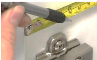
**STEP 1:** Mark how far back you want the slides to be. We recommend 80mm from the cabinet edge to the first screw hole. Place the slides in position before drilling hole to
