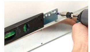
**STEP 4:** Use a level to mark the back hole. Drill hole & screw in the back end of the slide. 3 screws for each slide are sufficient.
