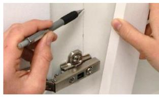
**STEP 2:** Use a ruler or baton to draw a straight line up the cabinet, this will give you a consistent set back when you install the upper baskets if installing more than one.
